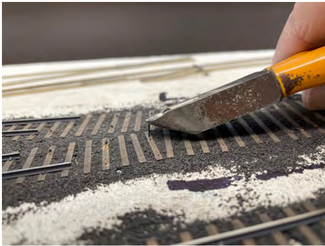
The first step was pulling up the spikes and rail as needed. I have some old, mangled rail nippers I use for spike removal.
