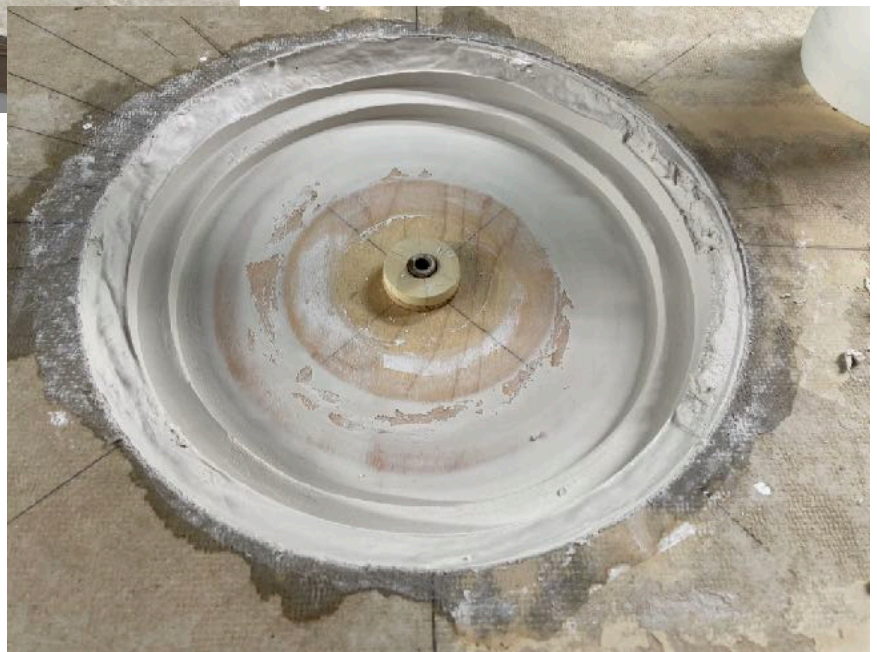
Left: Here is the wet plaster ready to be slopped into place and formed into the first attempt at contouring the pit.
