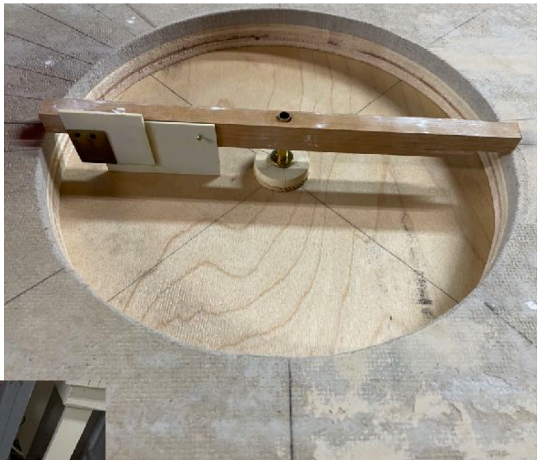
Above: This is the forming tool I built to get the contours of the turntable pit into the wet plaster. It rotates around a 1/4" brass tube fitted to the center bearings.
