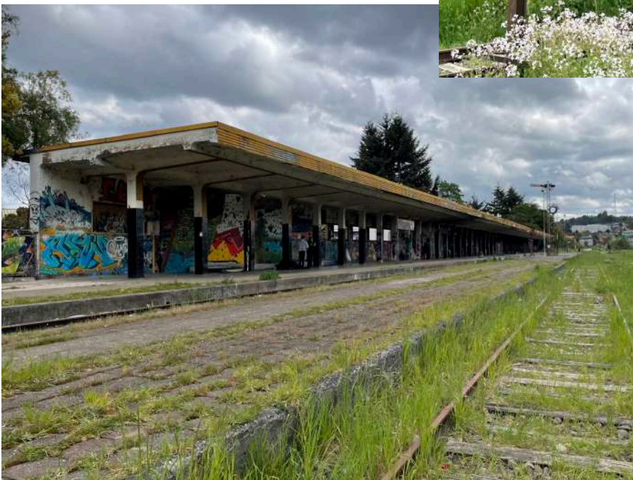
The station platform hadn't seen passengers in many years, but it had seen graffiti artists. It looks like there were more tracks at one time. Notice the semaphore in the background.
