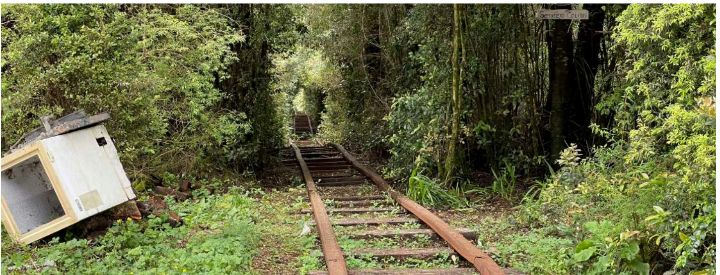
The square tubing rails of the home made railroad on Chiloé trundle off into the temperate rain forest.
