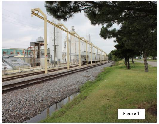
The Safety Rail is still standing and we felt is an important and prominent feature to be modeled. As you can see in the photo, the structure looks relatively simple. It is just a vertical beam, an angle, and a horizontal beam perpendicular to the railroad track supporting a long horizontal track
