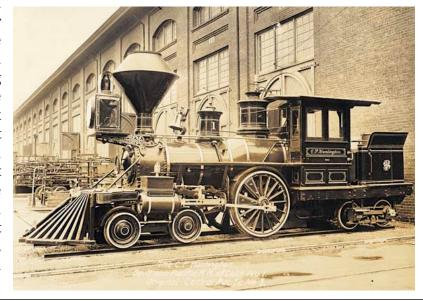
In 1863, a sister engine, the <u>T.D. Judah</u>, was built by the Cooke Locomotive Works for a railroad which was unable to pay for it and was purchased by the <u>Central Pacific Railroad</u>. This locomotive was rebuilt to a <u>4-2-2</u> wheel arrangement in 1872.
