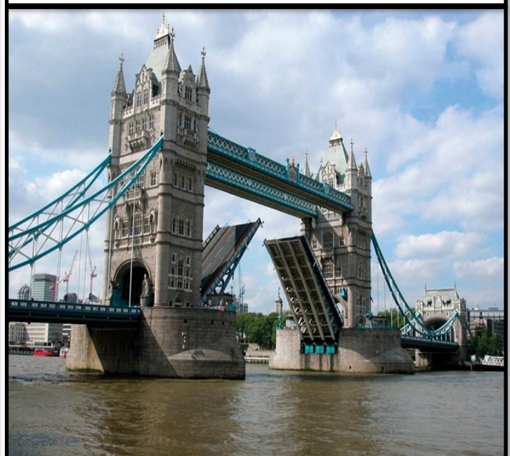
Bascule Tower Bridge. This is a vehicle bridge, but could also be a rail bridge. Photo from https://www.britannica.com/technology/bascule-bridge
