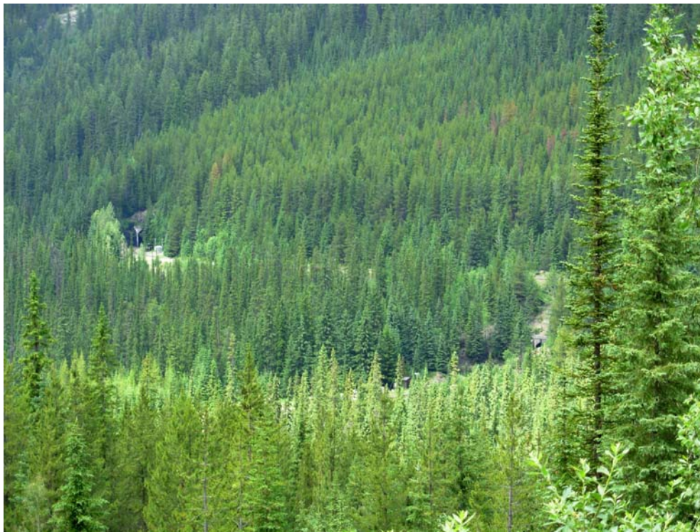
CP Rail's Lower Spiral Tunnels as seen from the viewpoint along the TransCanada Highway
