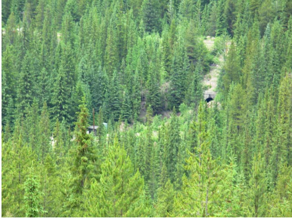
Lower portal, Lower Spiral Tunnel
