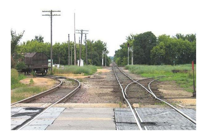
A junction or interchange location could also be created by two railroads operating "side by side" in a community. In this case, a track design needs to be created to allow the movement of cars between the two railroads, even though there are no crossing or diamond.
