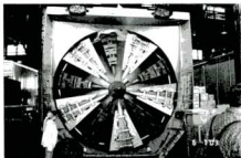
This view of Rotary 900082 shows the blades of the Rotary. The rotary support cars can be on each side of the rotary as it sits in the Roundhouse in Cheyenne.
