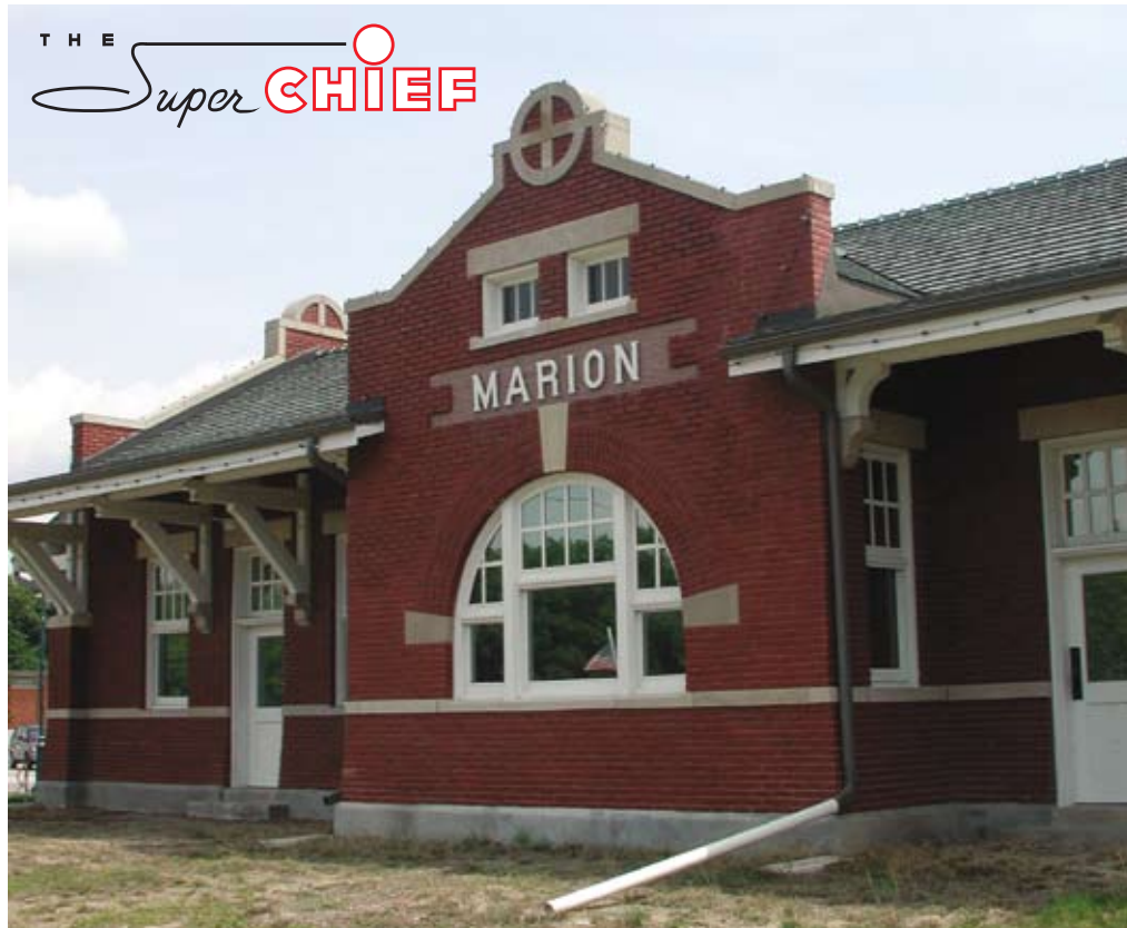
ABOVE: The southern face of the structure had the operator's window-office. Originally, a train order signal was controlled from this office, allowing the operator to stop a passing train for cargo, mail, or passengers. Robert L. Priest, photo
