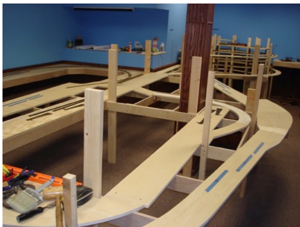
Pic 7: 11/19/15 - Sub-roadbed over frame construction begins using 3/4" solid core plywood.
