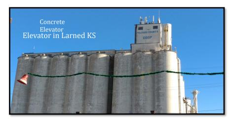
longest physical life. Concrete elevators come in many designs and configurations. Older concrete elevators consist of a head house, galley, tunnel, numerous bins. interstices. work areas. elevator shafts, etc. Newer concrete bins are being designed as free-standing with structures external elevator legs.
