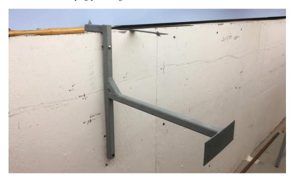
The L-girders in the front rest on the brackets and are bolted to the flanges.
