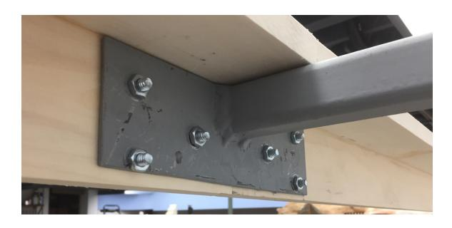
The L-girders against the wall were leveled with the front L-girders and attached with Tapcon concrete screws. They required shims to fit against my crooked walls.
