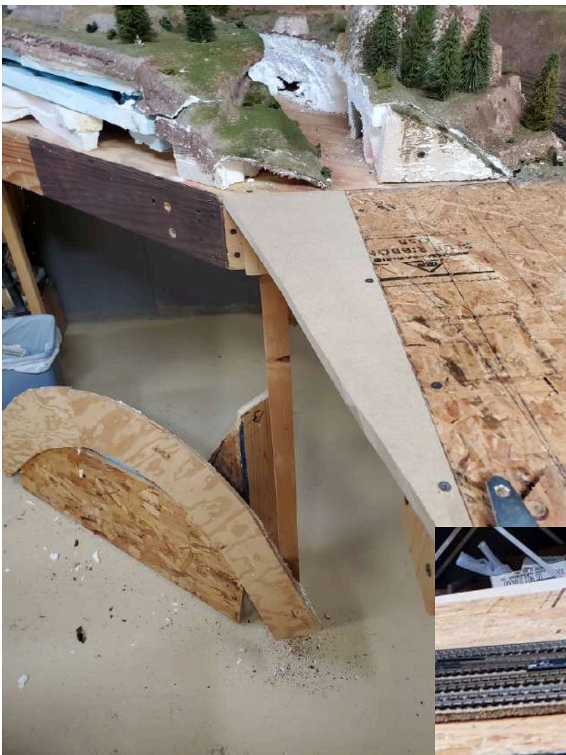
A piece of Homasote was cut to fill in the uneven edge between the hinged end and the unhinged end and to serve as a scenery base.
