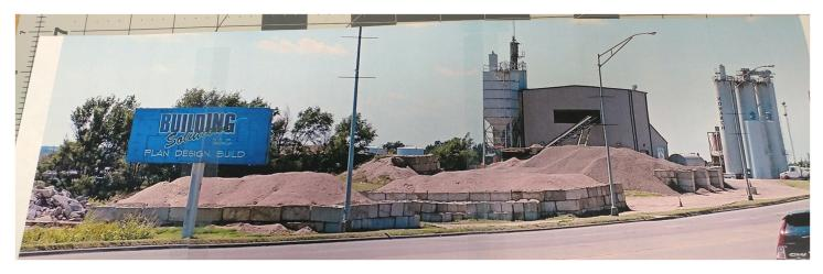
(Below) The original scene featuring a scale reduced Walthers HO-scale Cement plant. The silos on the right side are scratch-built and will remain to accept the cement powder arriving by rail. The rest of the structures will go.
