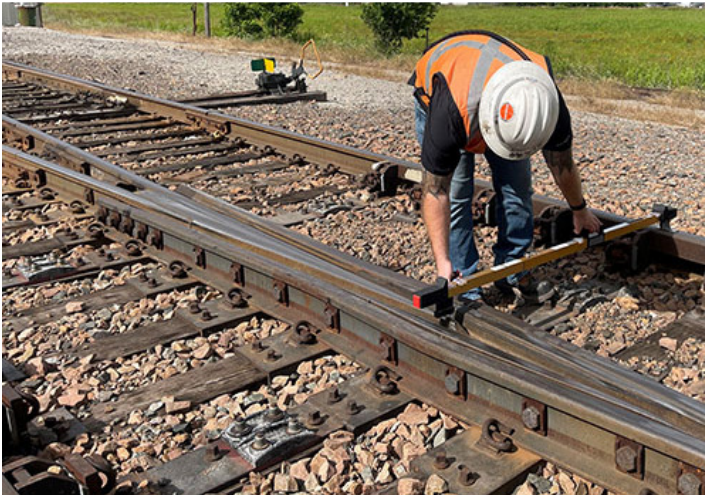
Cunningham measuring the distance between the rails using a track gauge
