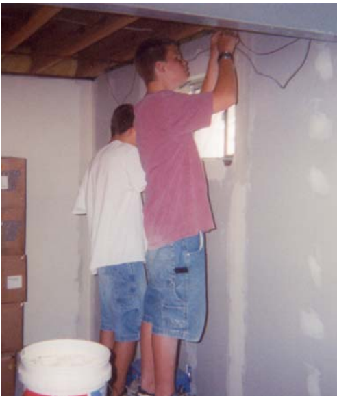
Photo 3: About ¾ done with the perimeter walls. Andrew Hoener, a local teenager with an interest in trains, is stapling telephone cables to the joists. Mark Rollins, another local, is taping joints in the background.
