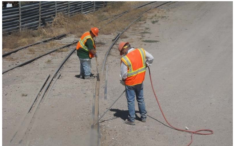
(Picture 4) Particularly on dirt or sand roads, road traffic carries the sand into the tracks. (Kelly Chopp Photo)
