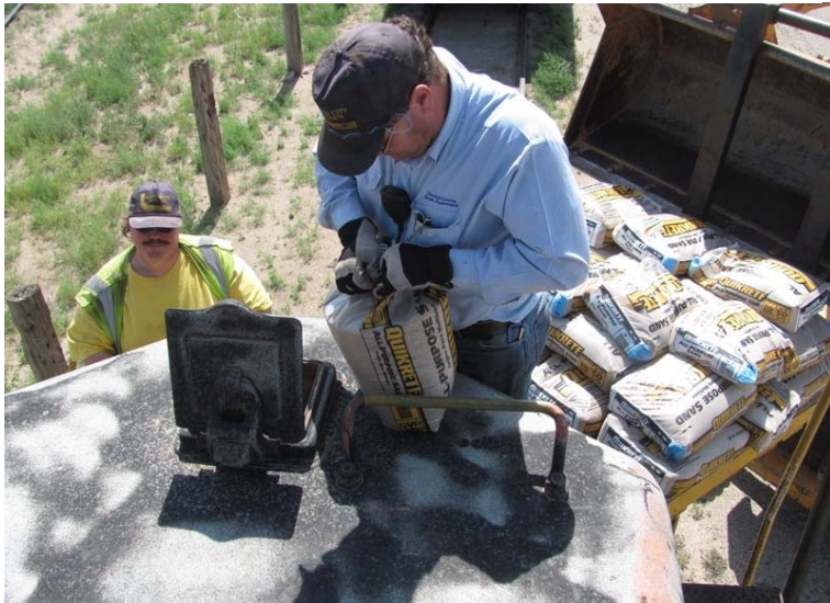
(Picture 2) The sand hatch is open, and bag by bag the locomotive gets it's load
